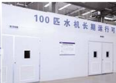
100Hp Long-running reliability lab (water) 150Hp Long-running reliability lab (fluorine)
